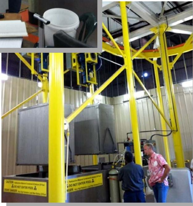
Pa'ina Irradiator post-construction – completely built out former agricultural building with irradiator equipment installed and operational.
